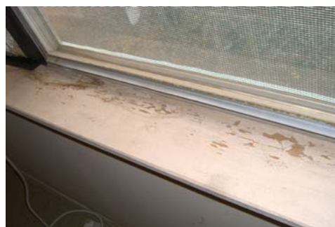
Window sills show water damage because windows are old style
