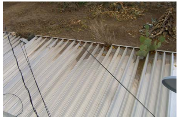
Those are plants growing on top of the patio roof
