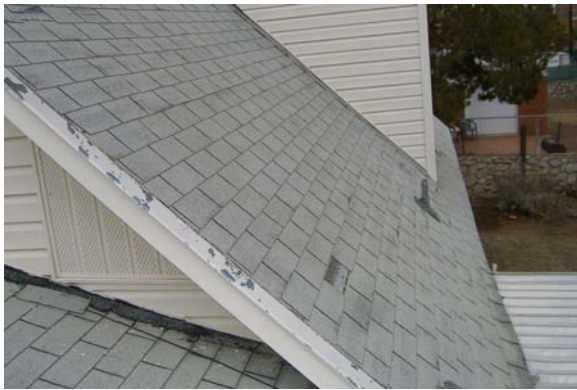
Photos showing other areas of the roof with missing shingles.
