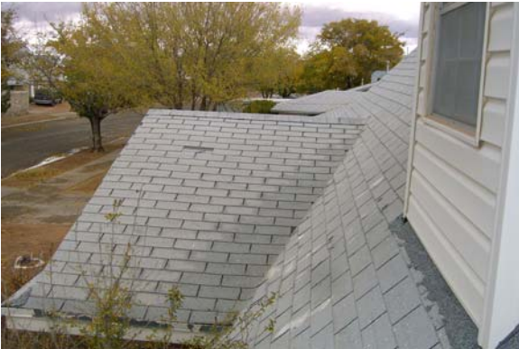
Photos showing other areas of the roof with missing shingles.
