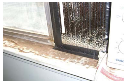
Window sills show water damage because windows are old style
