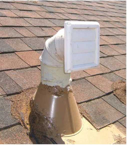
Example of back draft damper for proper dryer exhaust.
