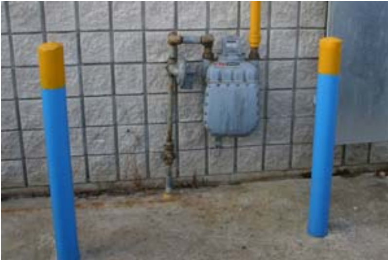
Example of barriers to protect gas meter.
