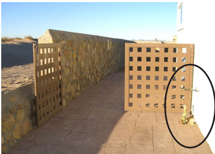
Your gas meter is in the driveway where it can be hit by a car.
