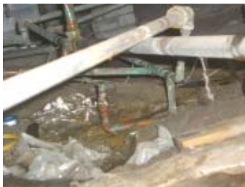
Fixtures are corroded and are not functioning
