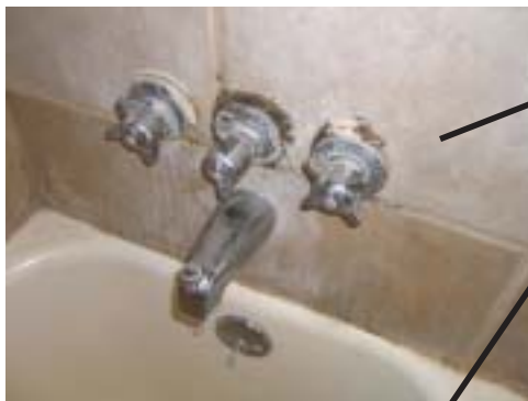
Fixtures are corroded and are not functioning
