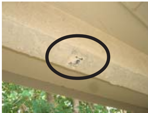
Water damage on the bottom of the patio fascia area
