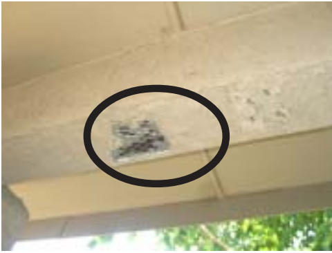
Water damage on the bottom of the patio fascia area
