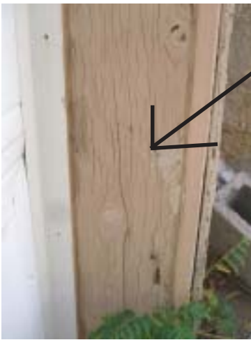
Water damage on the bottom of the patio fascia area
