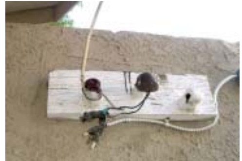
On the right is the wiring for the garage on the outside wall. It should be in conduit and should have junction boxes to protect the wiring and to protect against shock.
