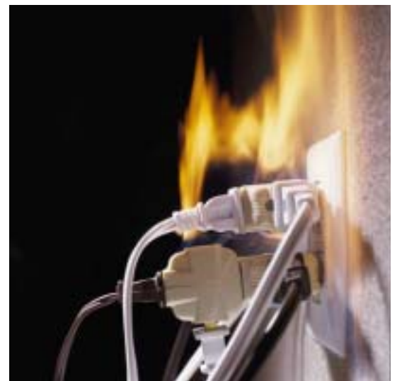
An overloaded outlet is a major cause of household fires.
