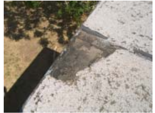
These three photos are of the rolled roofing over the patio. It was not replaced when the new roof was put on in Feb. 2011. It is in very poor condition.
