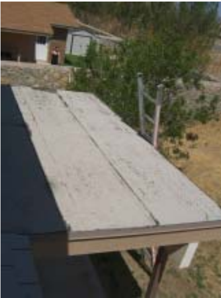
These three photos are of the rolled roofing over the patio. It was not replaced when the new roof was put on in Feb. 2011. It is in very poor condition.
