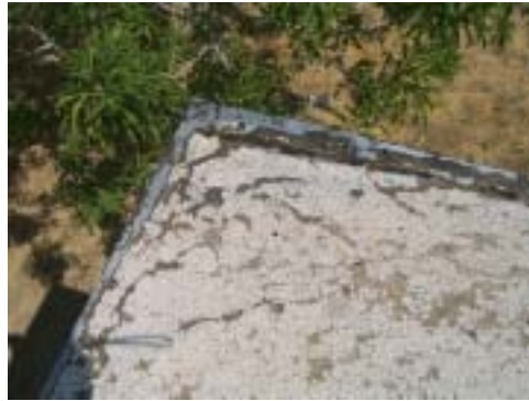
These three photos are of the rolled roofing over the patio. It was not replaced when the new roof was put on in Feb. 2011. It is in very poor condition.
