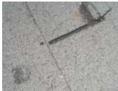
The shingles over the garage were a little beat up when they were installed. This will shorten the life of these shingles in this area.
