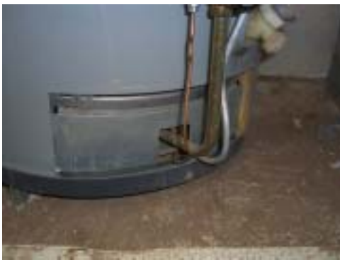
There should be a cover plate in this area.
