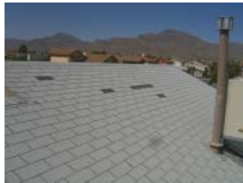
These are photos showing sample areas where shingles are missing.
