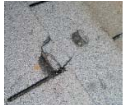
The shingles over the garage were a little beat up when they were installed. This will shorten the life of these shingles in this area.
