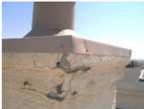
Another area of stucco damage on the chimney chase.
