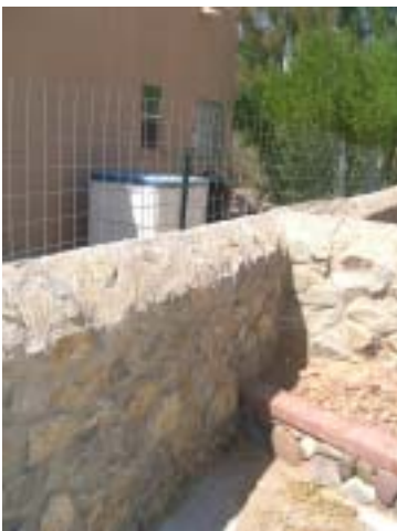
Left photo shows climbable wall. Center photo is a gate that is not self-closing. Right photo shows the wall not being 48" high on the right hand side.
